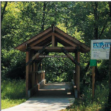
A multi-use trail could provide bicycle facilities in the floodplain
