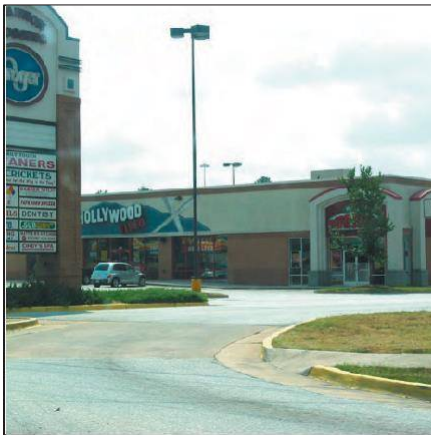
Curb cuts at each and every business create unsafe conditions
