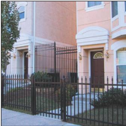
Taller fences are provided between buildings, while lower fences with gates are along the street.
