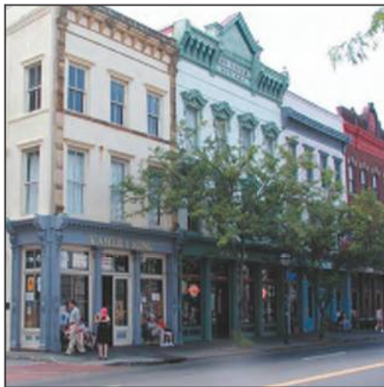
These historic commercial structures in Charleston create a pleasant streetscape
