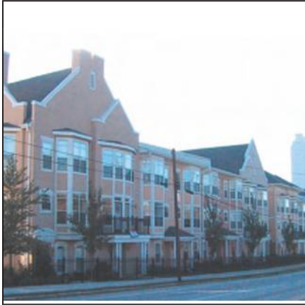
A small low fence surrounds these townhomes, while the buildings themselves create a barrier to internal areas.
